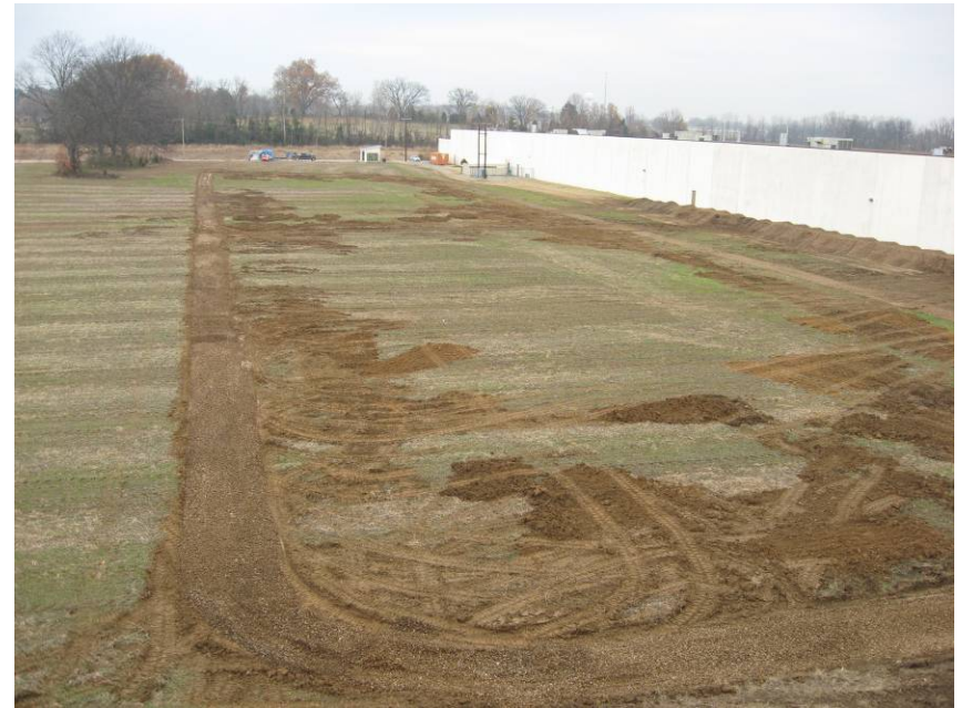
The Walking Track is under construction.
